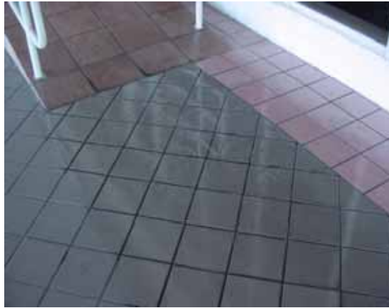
Polished & Quarry Tile Walkway Grand Hotel & Condo-Miami
