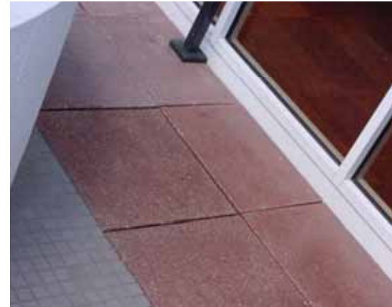
Tinted Concrete Grand Hotel – Pool Deck
